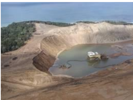
ABOVE. Richards Bay Minerals dune mining operation on KZN North Coast.
